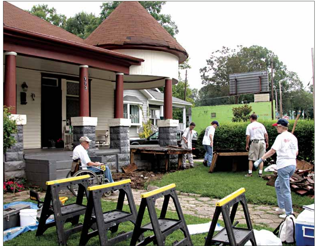
Demolition begins at 773 Pryor Street
